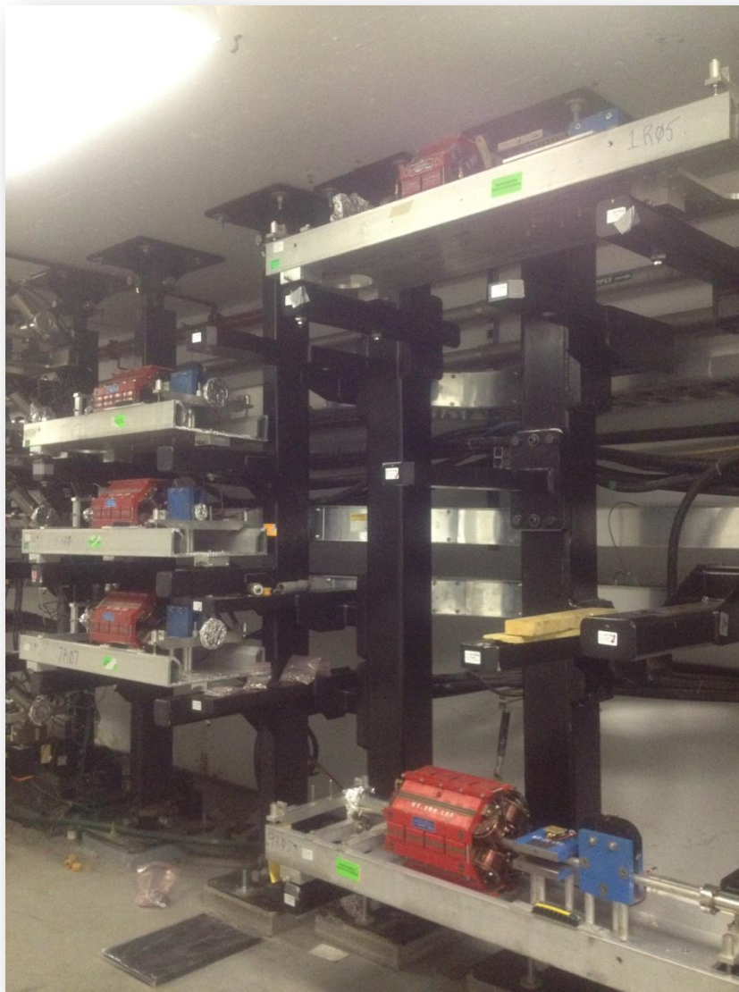
Girders installed in 1R
